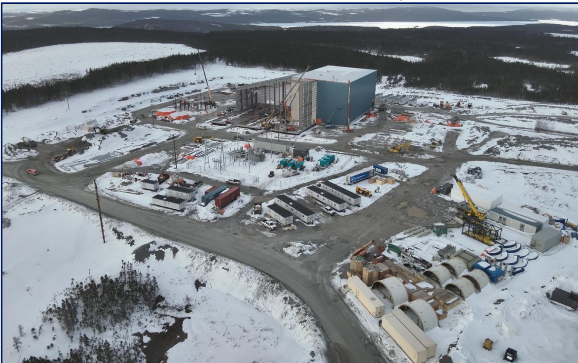
Valentine Gold Mine Plant Site as at March 23, 2024
