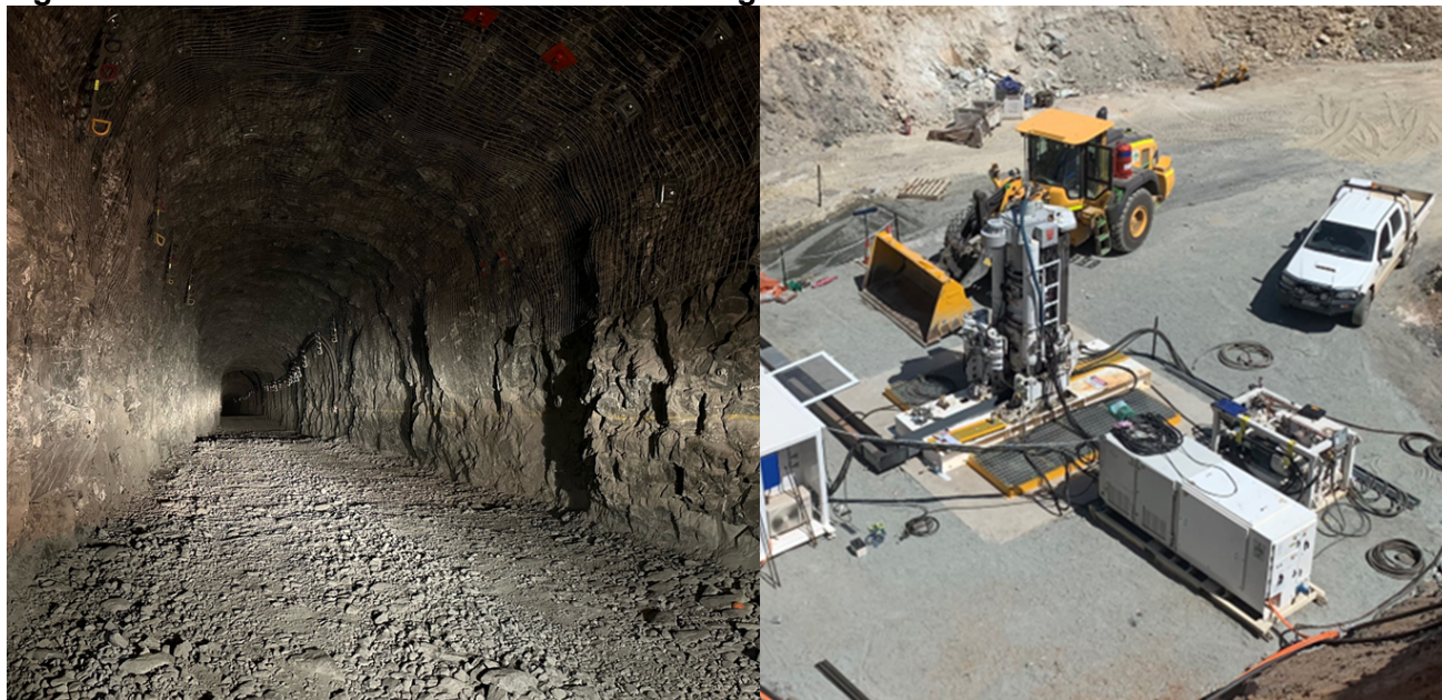
Figure 2: Beta Hunt second decline breakthrough and vent raise installation
