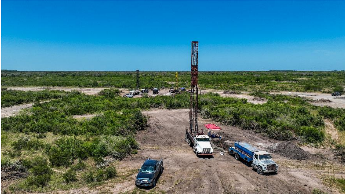
2023 Drilling program at Burke Hollow ISR Project, South Texas
