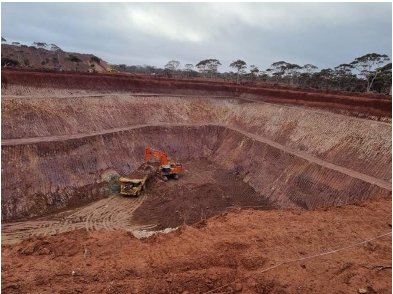
Figure 3: Aquarius Mine box cut
