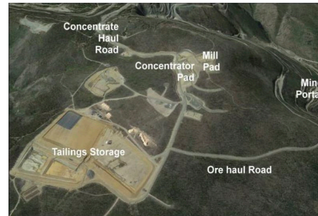
A large part of the mining area has already been built. (Source: eCobalt Solutions)
