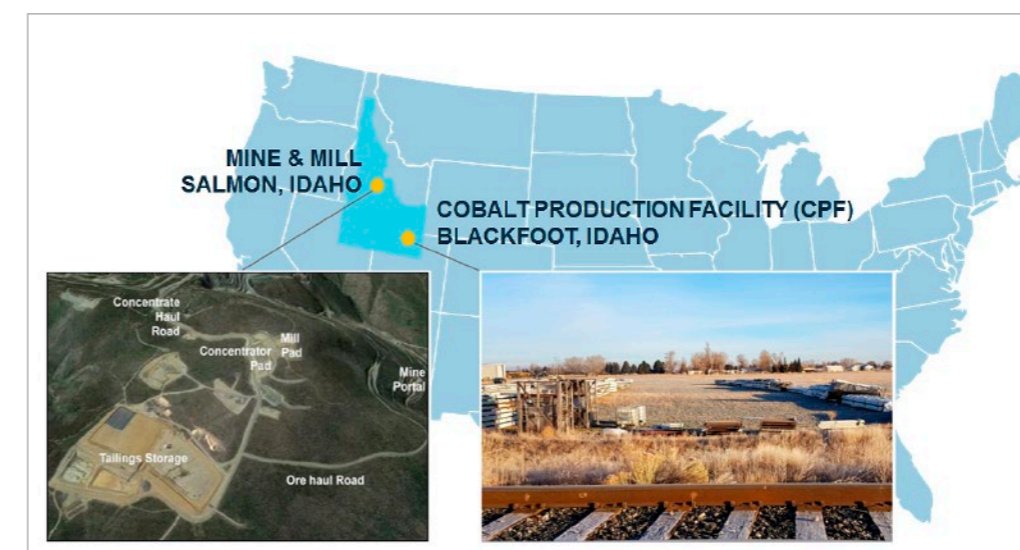
A large part of the mine installations is already in place or in the process of being built. (Source: eCobalt Solutions)
