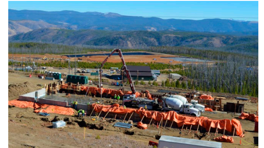
Concentrator Building Construction (Source: eCobalt Solutions)
