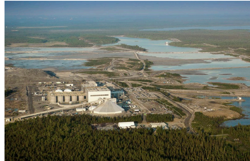
Canadian Malartic, currently the largest Canadian gold mine. (Source: Osisko Gold Royalties)
