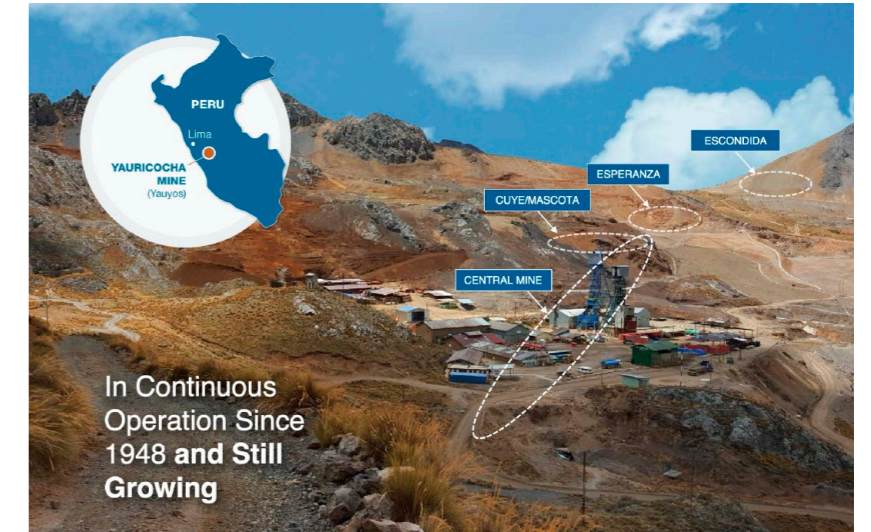
Yauricocha Mine – in continuous operation since 1948 and still growing (Source: Sierra Metals)
