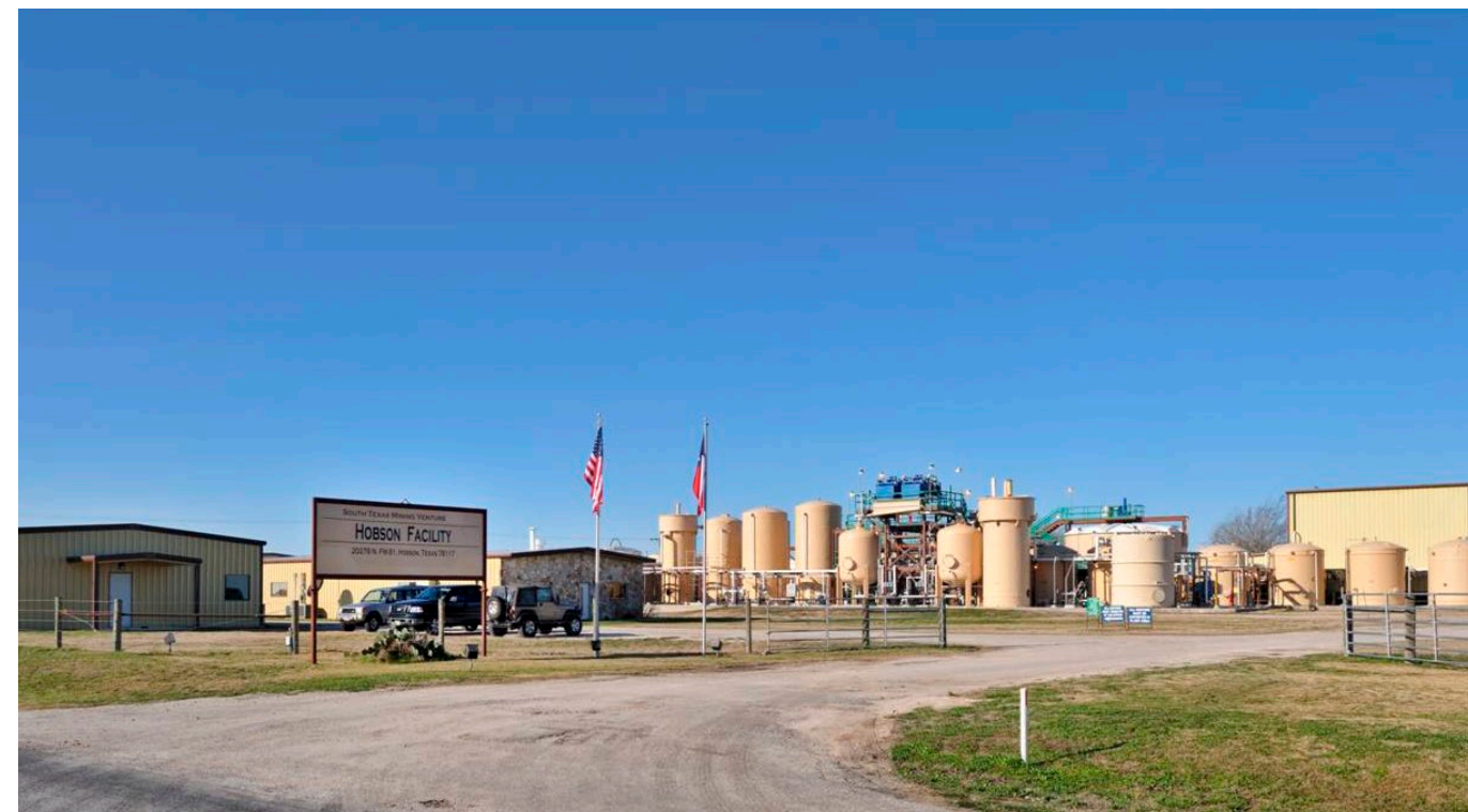
The Hobson production facility has been completely renovated and is state of the art. (Source: Uranium Energy)
