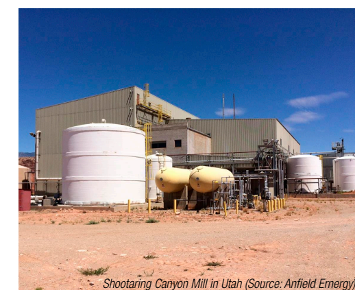
Shootaring Canyon Mill in Utah (Source: Anfield Energy)
