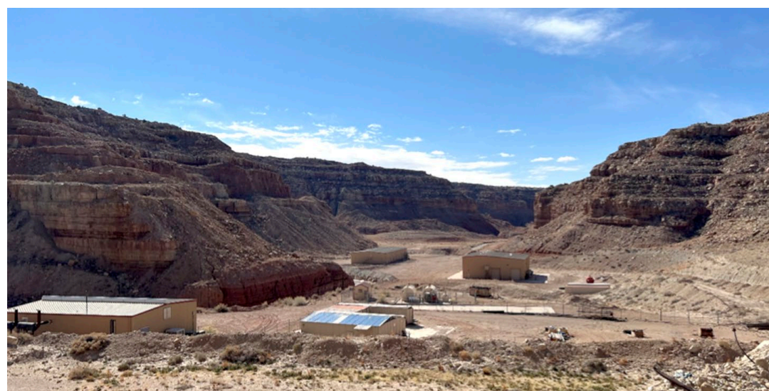
Significant Infrastructure at the Past Producing Tony M Mine, Utah (Source: Consolidated Uranium)
