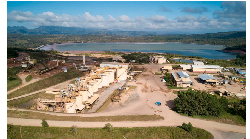
The La Libertad processing plant can process about 2.25 million tons per year (Source: Calibre Mining)
