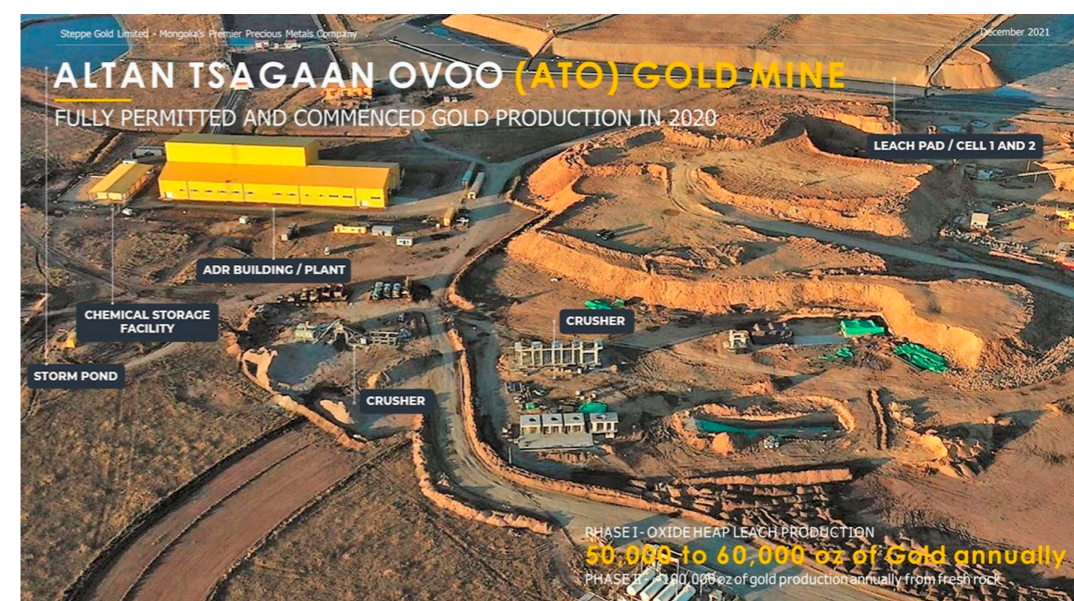
ATO Gold Mine Infrastructure Expansion (Source: Steppe Gold)
