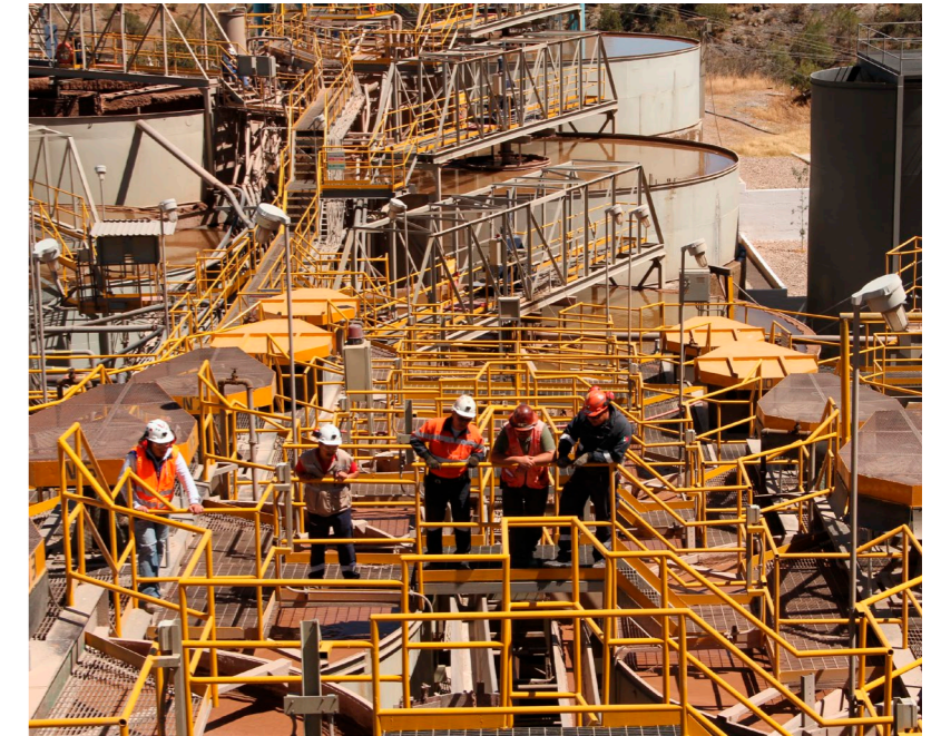
Guanaceví is the first and highest-grade silver mine (Source: Endeavour Silver)
