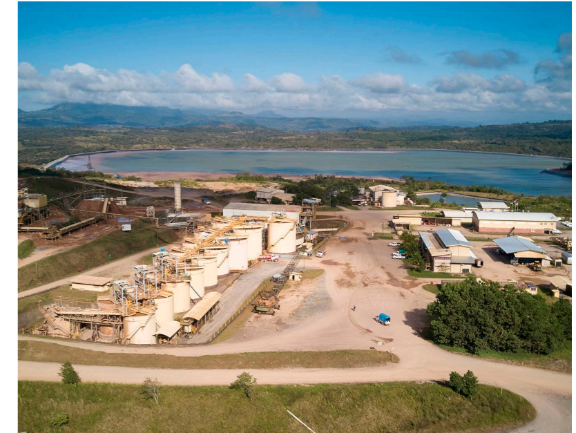
The La Libertad processing plant can process approximately 2.25 million tons per year (Source: Calibre Mining)
